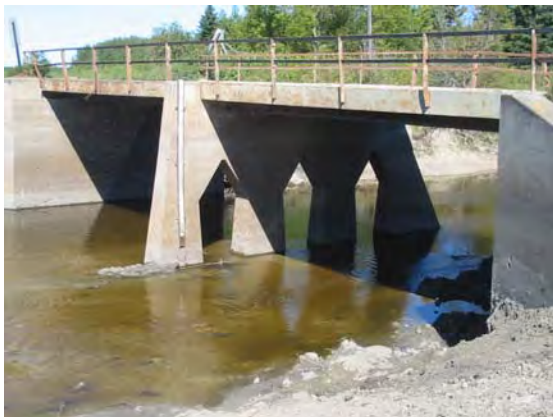
Silt Removed, Marshall County Road #7 Section 32 East Valley Township
