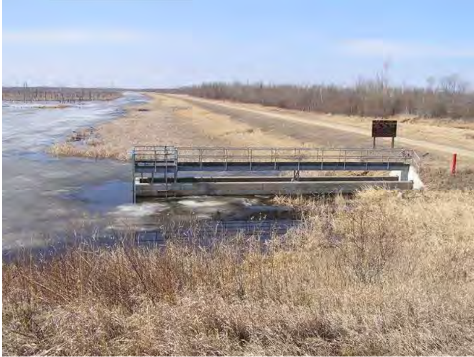
North Pool - Gated Principal Outlet Structure
