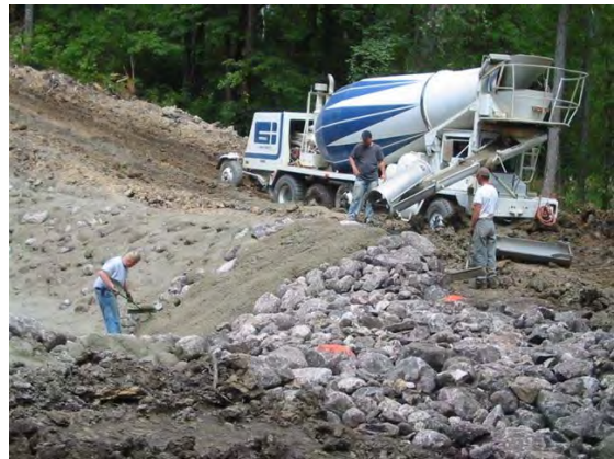
Grouted rock chute at outlet.
