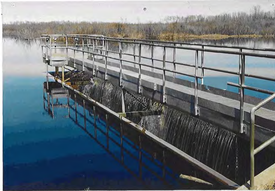
South Pool - Gated Principal Outlet Structure
