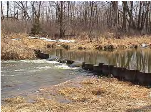
Sheet Piling Weir with 2 adjustable stoplog bays
