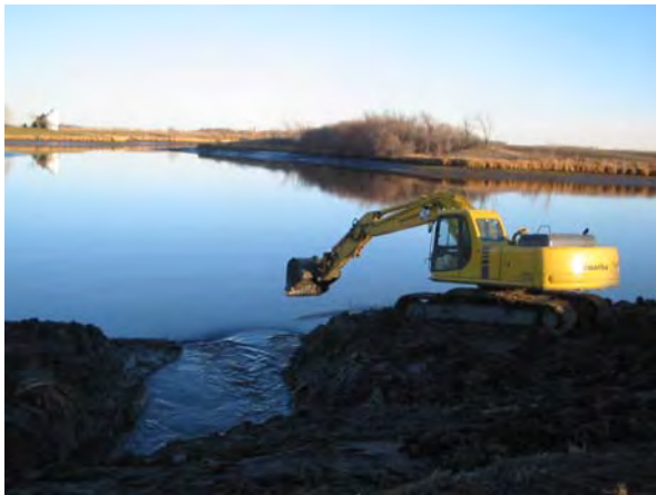
Excavation for Pool Drawdown
