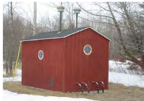
Air compressor house for bubbler system
