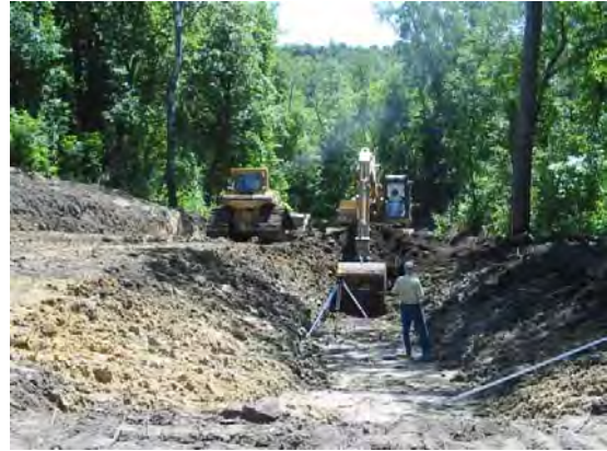
Location and excavation for rock chute at outlet of ditch.
