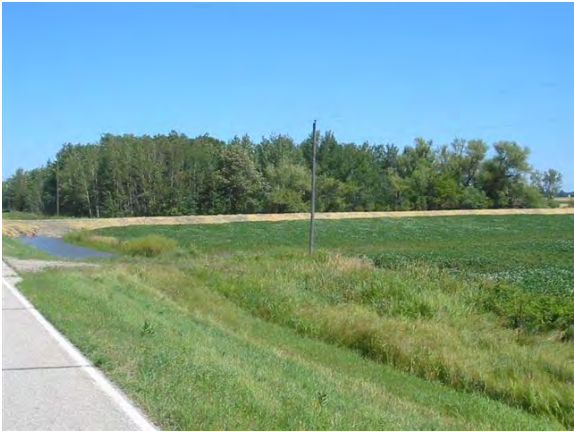
Ken Grundhaus ring dike construction, located in Section 18, Agder Township, Marshall County.
