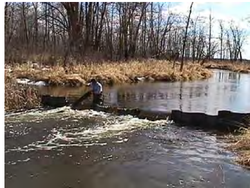
Removing stoplogs to manage lake level
