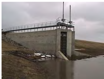
Principal outlet structure hydraulic gate operation
