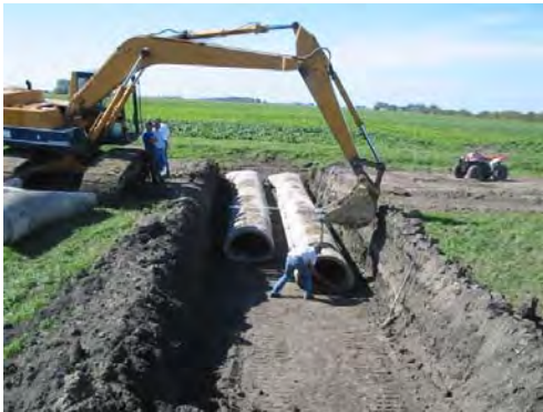
Richard Stengl ring dike construction. Located in Section 30, Tabor Township, Polk County
