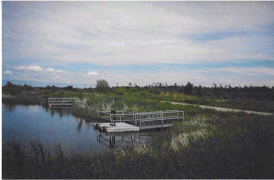
Gated Principal Outlet Structure
