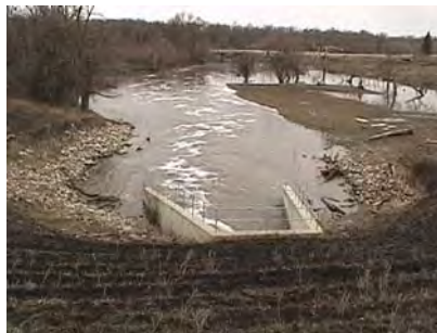
Looking downstream from outlet structure
