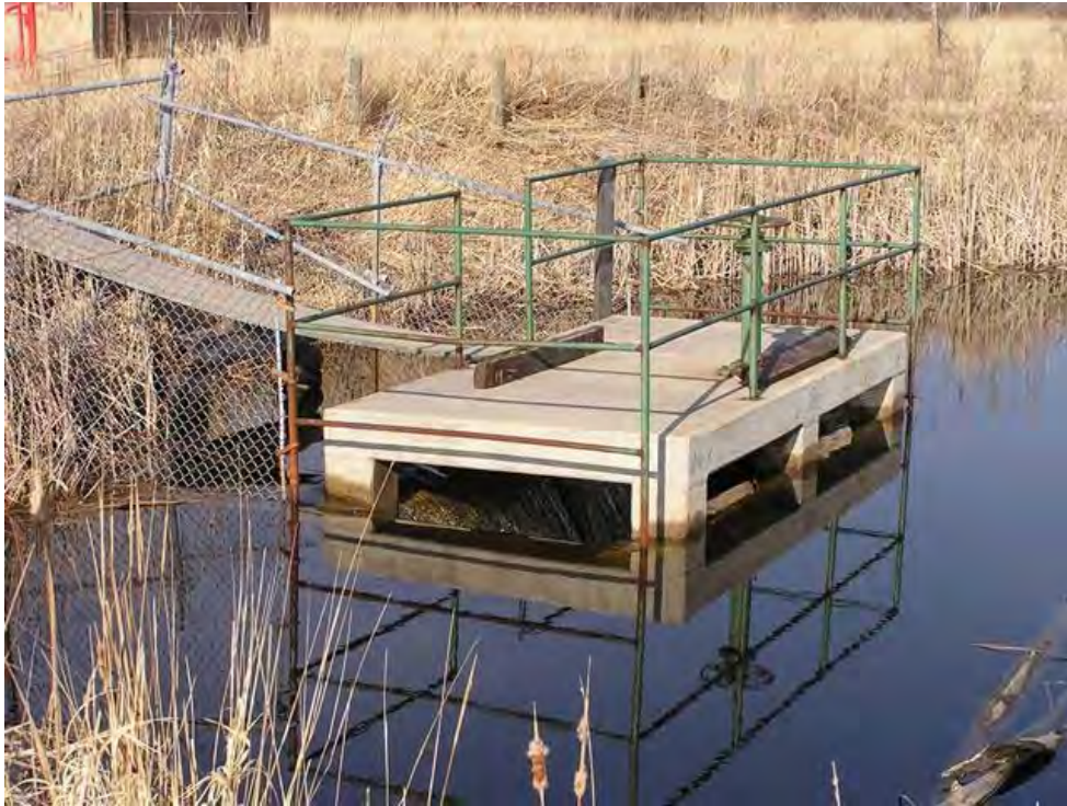
Lost River Impoundment Outlet Structure
