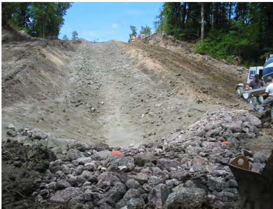
Grouted rock chute at outlet.
