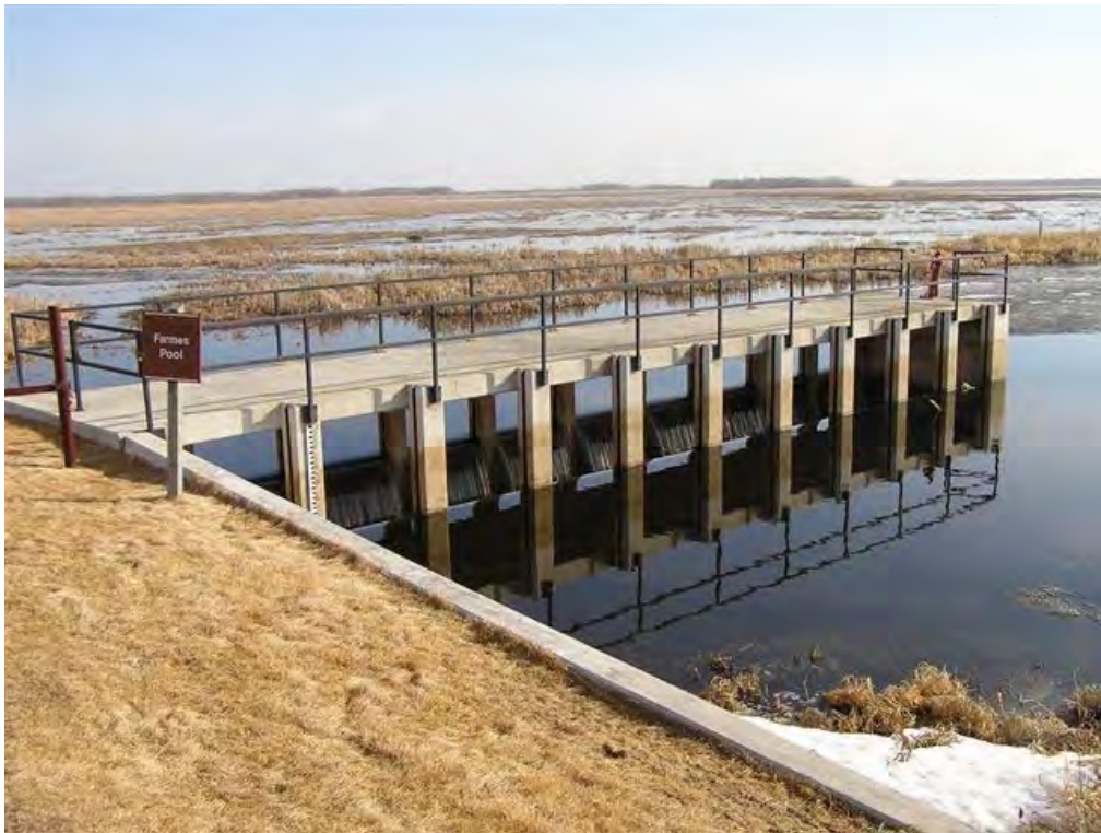
Stoplog Outlet Structure
